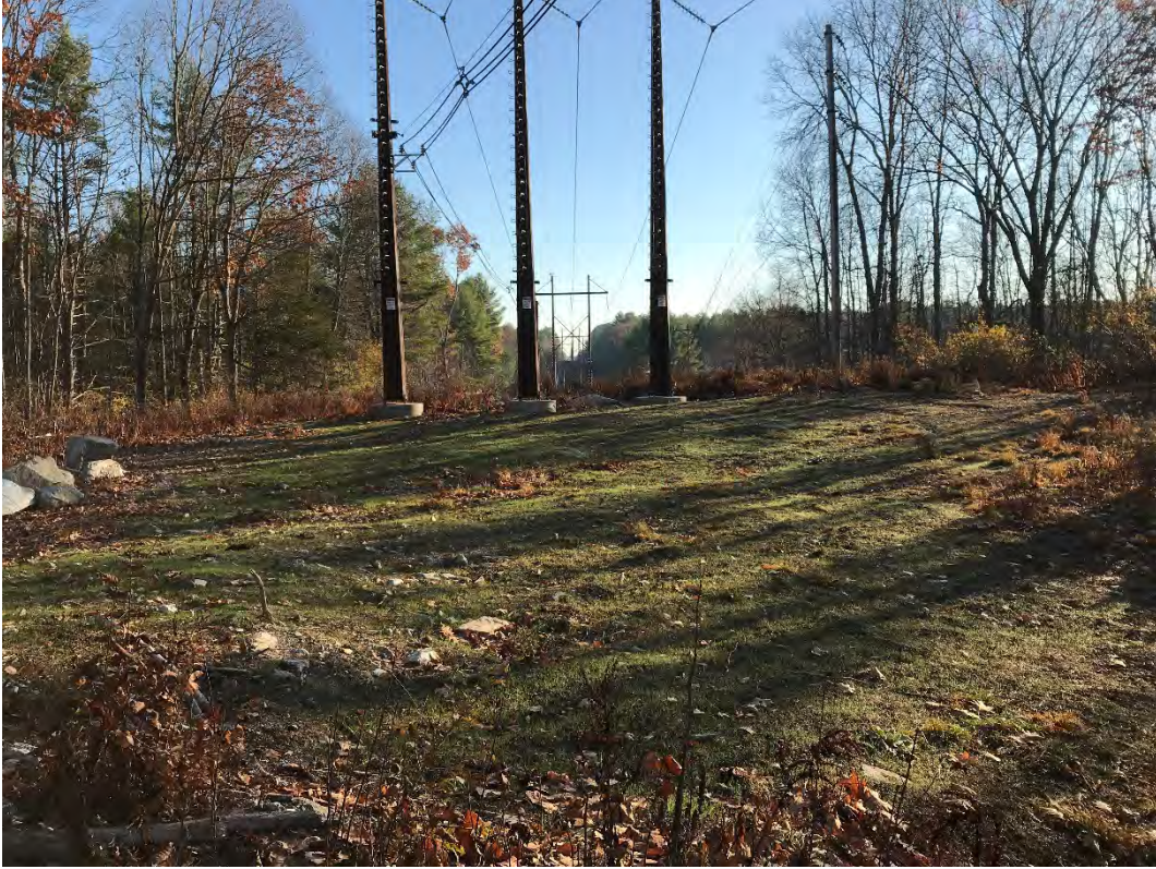
Fig 9: Str. 58 work area. Viewing east. (11-10-20)
